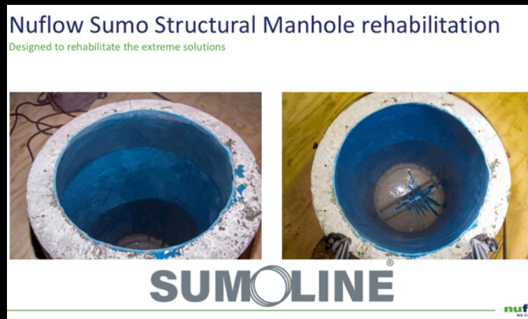
Structural fit for purpose man hole rehabilitation
