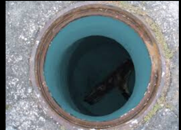
spray epoxy structural relining
